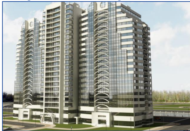
Building No.5A – Antares building
