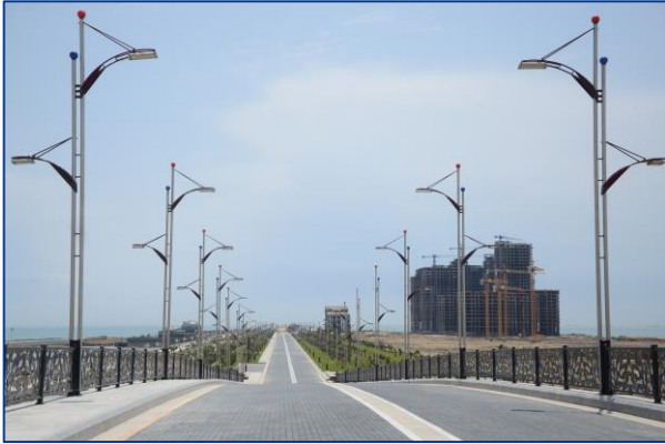
Roads with the granite pavements
